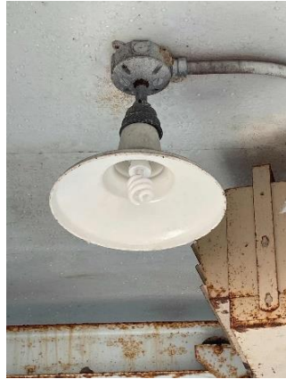
Chlorination Pumphouse: CFL Fixture
