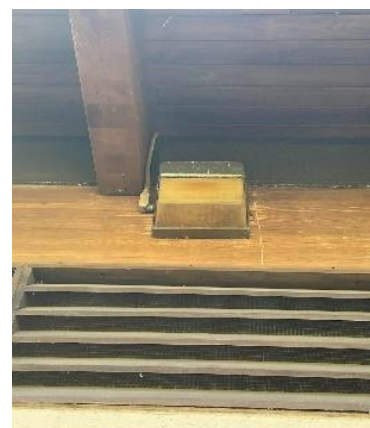
Bathhouse Shower: High-Pressure Sodium Exterior Fixtures
