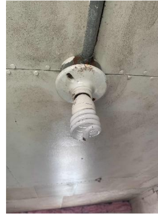
Bathhouse Pumphouse: CFL Fixture
